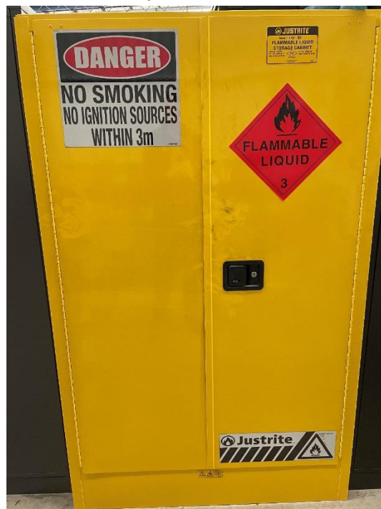
Figure 28: Small package Flammable Liquids Cabinet – Location workshop
